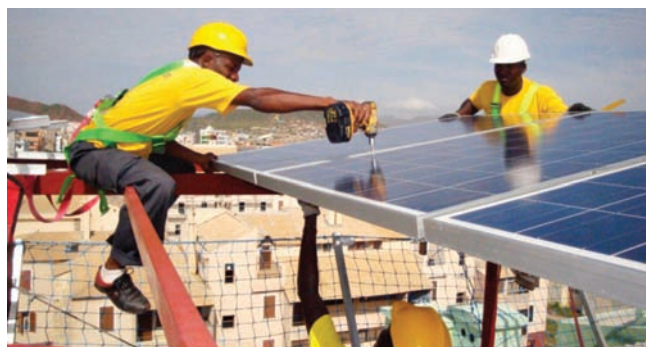
Installation of the Solar PV system at ECREEE Headquarters
