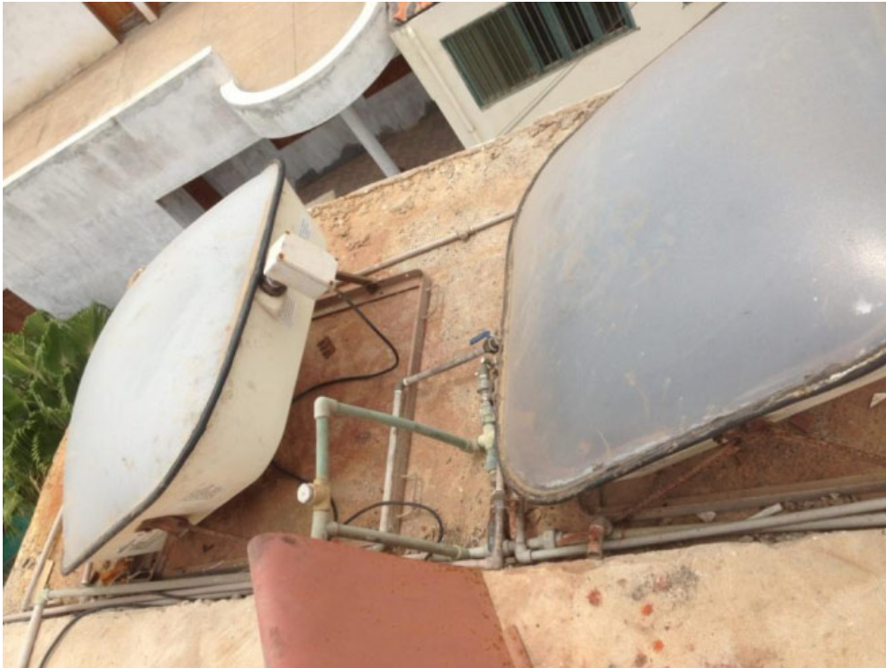
Figure 4 – DISCOTERM (technical data annexed) 135 liter direct type solar water heater (details in annexes)
