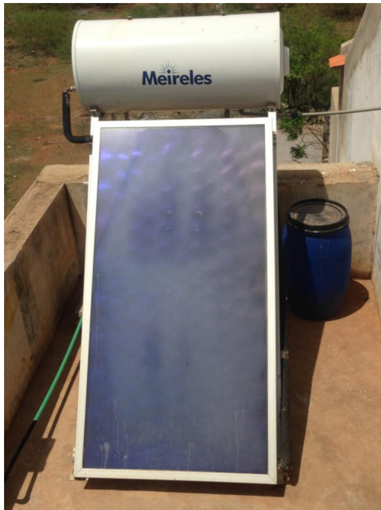
Figure 17: Thermosyphon system found on single family house of 4 persons with storage of 190 liters. On the 13 of September, 2015 at 13:50 local time a temperature of 69.2 °C was recorded from the outlet of storage tank. Positioning of the collector is not optimized (>45 degrees) because of lack of space.
