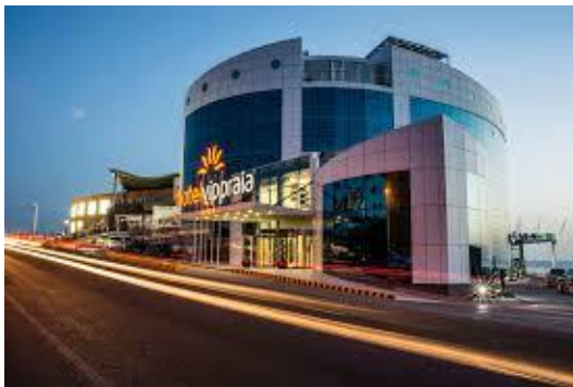
Figure 23: VIP PRAIA Hotel 79 rooms fitted with electrical hot water heaters, innumerable compression type AC units and all façades (west, south, etc.) made of glass.
