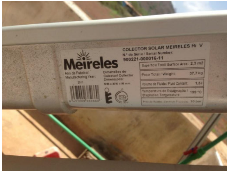
Figure 18: Parameters of collector shown in figure above. Storage tank for this system weights 83 kg (empty) and have capacity for 190 liters.
